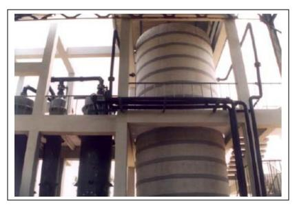
Fig 1. ISET Scrubber at KCPSIC Limited, Vuyyuru, Krishna District, Andhra Pradesh, India - for Biogas from Distillery Effluent Treatment Plant
