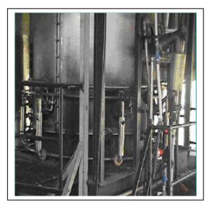
A specially designed pilot burner has been provided to prevent flame flash back during initial gas flaring period. This was extensively tested at the laboratory prior to installing at site.
