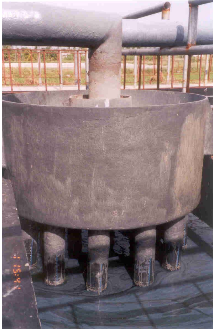
FEED INLET ARRANGEMENTS
