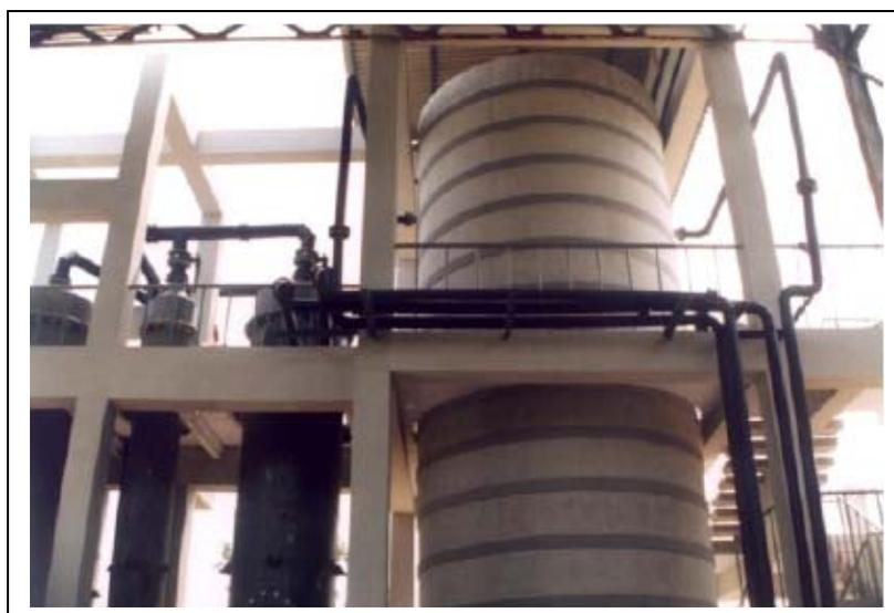
Fig 1. ISET Scrubber at KCPSIC Limited, Vuyyuru, Krishna District, Andhra Pradesh, India - for Biogas from Distillery Effluent Treatment Plant
