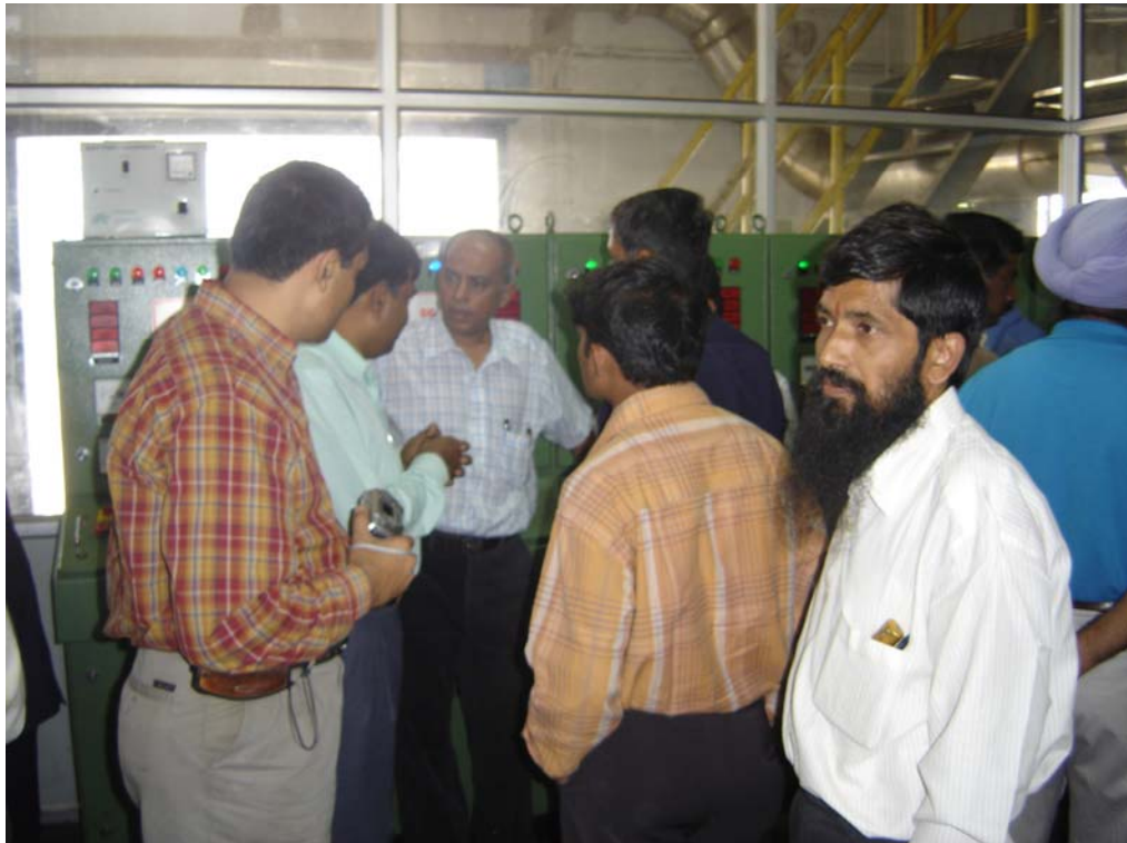
Control Room of Arashi
